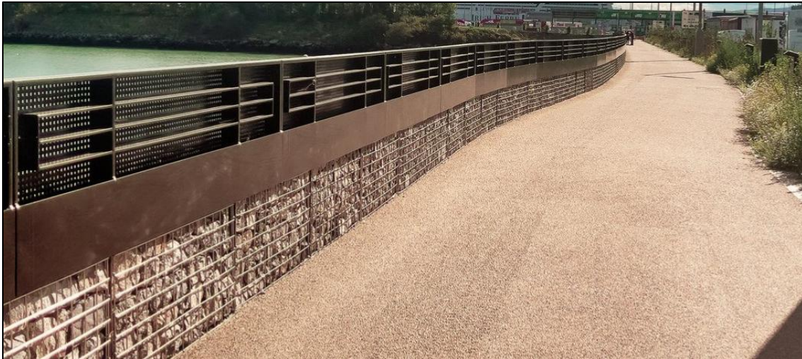
Plate 4 Low permeability perforated screening on the Dublin Port Greenway.
